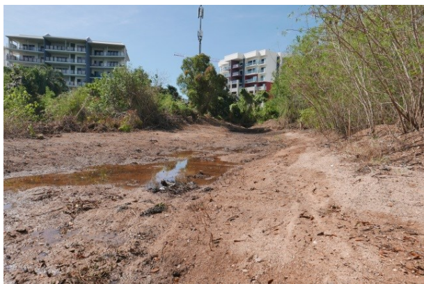
Figure 6. Old Phoenix Hotel drain de-silted, with minor shallow ponding
