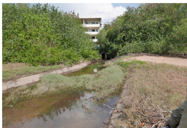
Figure 4. Sunset Cove drain blocked with vegetation
