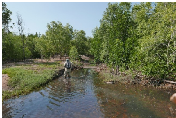
Figure 4. Sunset Cove drain blocked with vegetation
